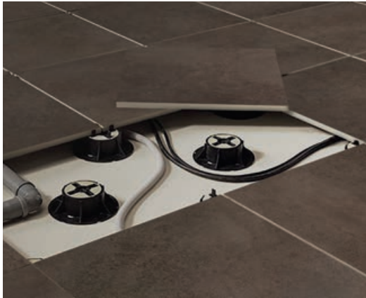
Laying as raised paving. Colocación sobreelevada.
